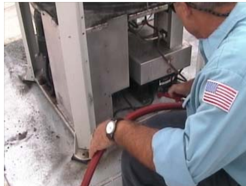
Figure 6. Wash the bottom shelf of the compressor unit
