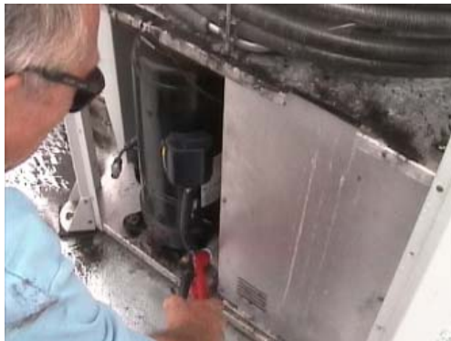
Figure 6. Wash the bottom shelf of the compressor unit
