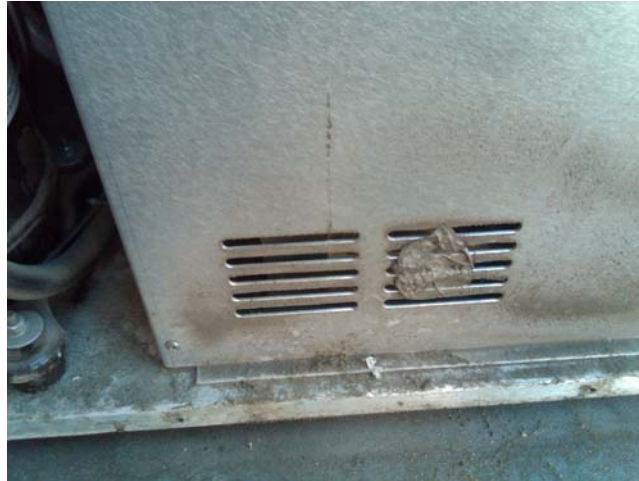
Figure 5. Remove any debris from the electronics bay ventilation louvers
