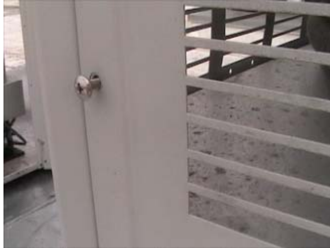
Figure 7. Start but do not tighten all of the screws holding up the side panels
